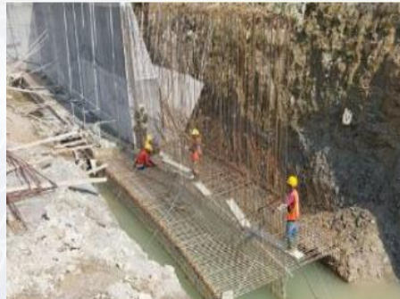
Sandtrap Install Rebar Footing
