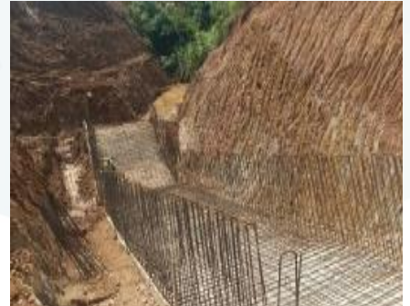
Install Headpond Rebar Flushing
