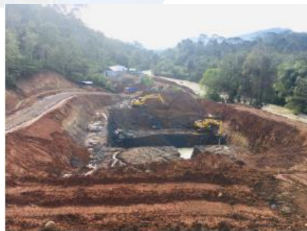
Power House Constructions
