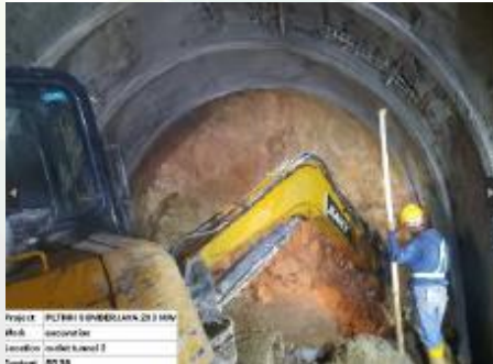
Tunnel Excavation Outlet, Pouring concrete cyclops,
