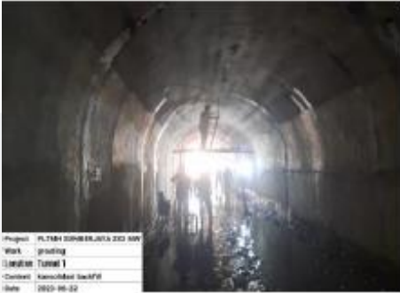
Tunnel Grouting Backfilling
