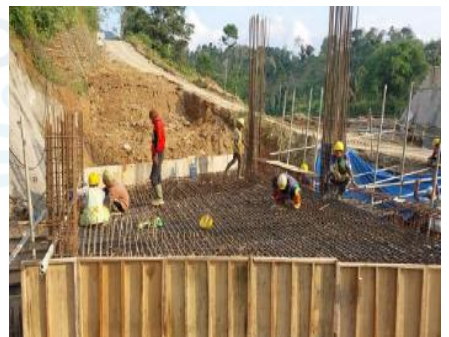
Install intake rebar and bekisting slab
