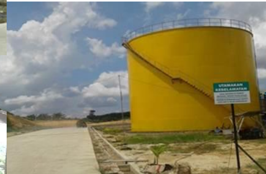
CPO Storage Tank
