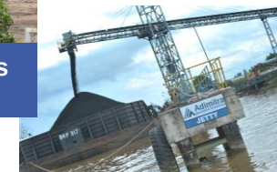
Overland & Barge Loading Jetty: Kecepatan loading 1.800 ton/jam
