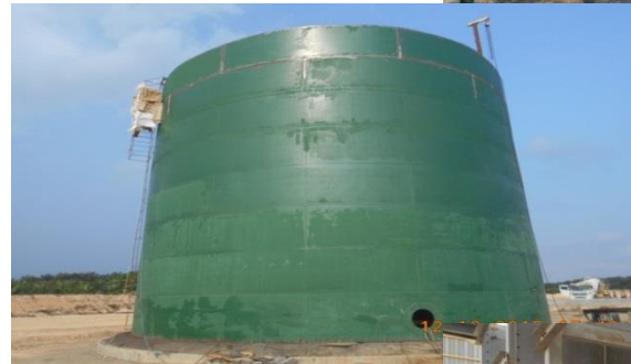
Oil Storage Tank
