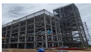
GLP Main Building Installation
