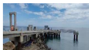
GLP Coal jetty construction
