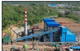
MCL Main Power House
