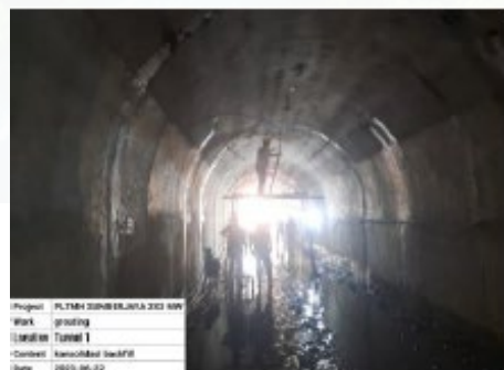
Tunnel Grouting Backfilling
