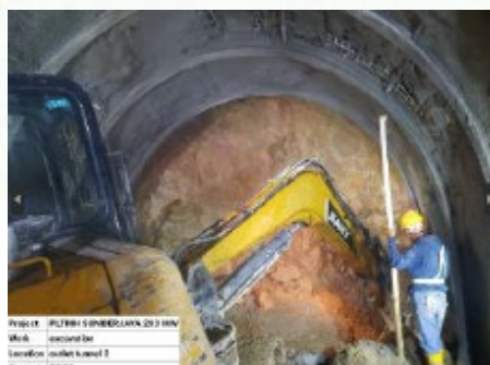
Tunnel Excavation Outlet, Pouring concrete cyclops,
